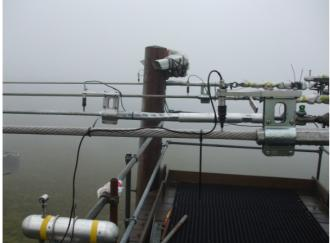
Fig. 3.3 Vibration monitors installed on all the conductors
