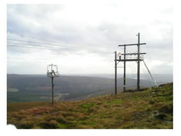
Fig. 2.1 The southern H-pole of the Deadwater Fell main test span and the rotating rig.
